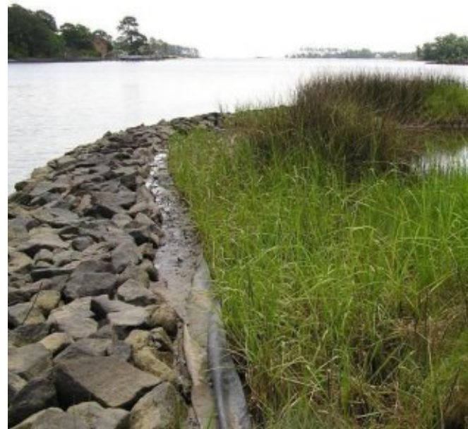
Example of using rock to protect adjacent coastal wetland. Credit, CCRM.
